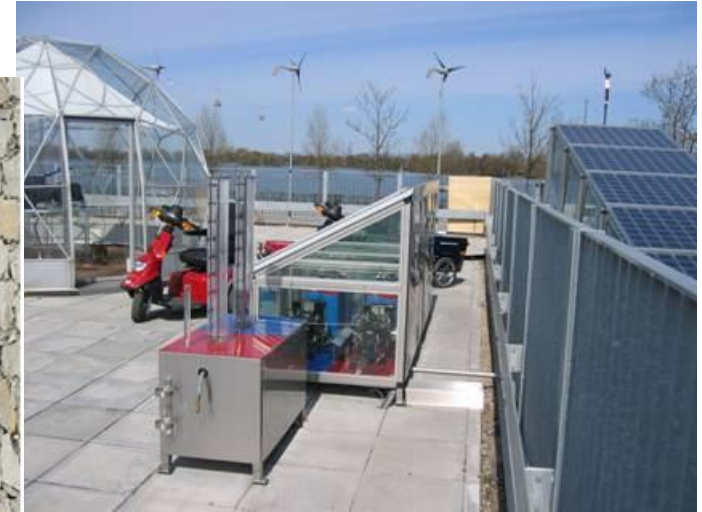
Electrolyser and Fuel Cell
